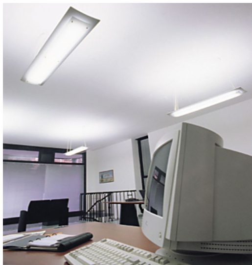
Figure 27 Lighting left on in an empty office
