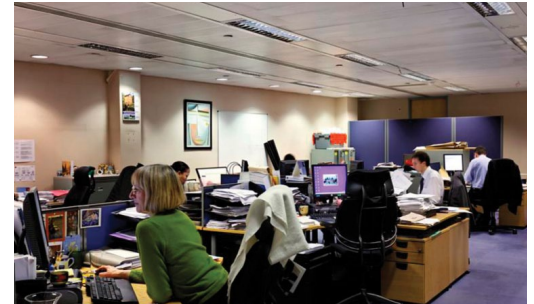
Figure 34 Poor LG3 application
