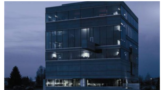
Figure 37 A well controlled office building with lights turned off at night
